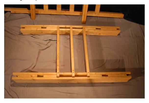
The top piece is made out of the 2"x6"s. Assemble the 8'x2"x6" boards and choose the two nicest of the sides these will be on the outside where most people will see them.
